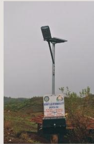
Solar Lamps in Adiwasi Area
